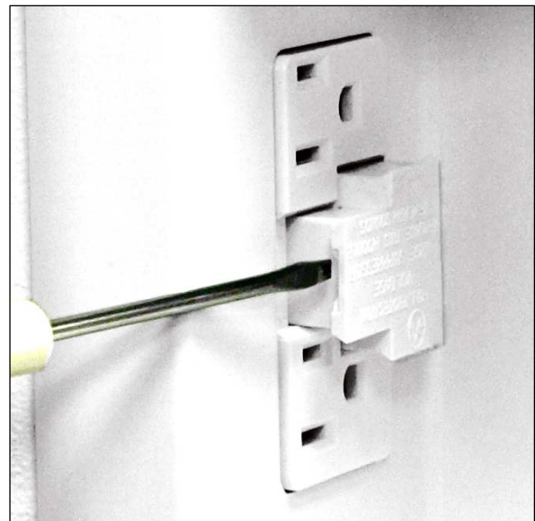
Removing the SurgeBloc® Module
